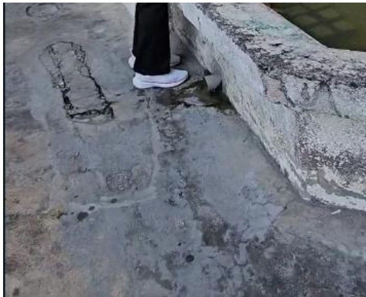
Figure 4: Condition area curing pond
